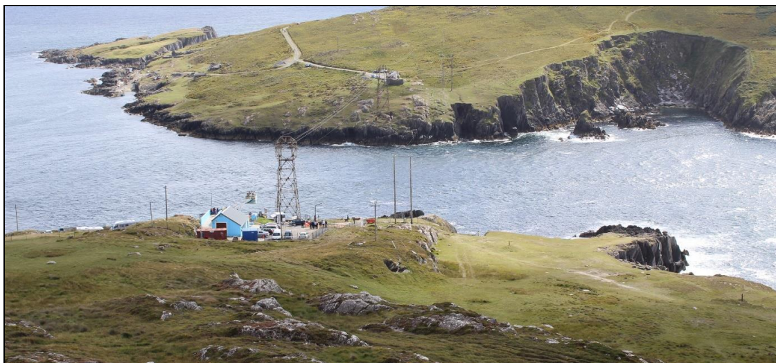
Plate 11.5 Steeply sloping topography towards cable car infrastructure on both sides of Dursey Sound
