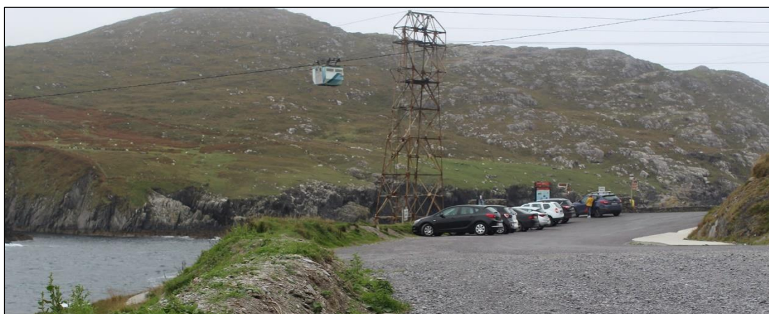
Plate 11.6 Car park along the access road to the cable car
